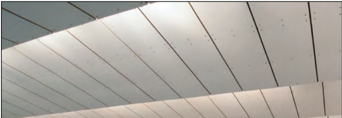
Baffle Fascia: When the ceiling baffles are shot repeatedly, the fascia can easily be replaced with the existing screws.
